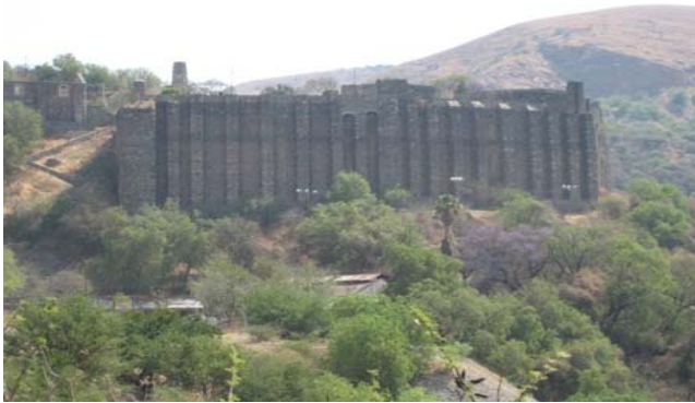
Picture 3. Shaft structure at Rayas Mine
