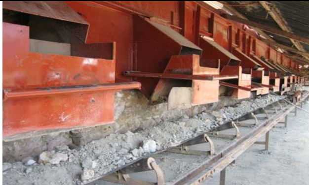
Picture 11. Multiple ore bins allow processing various feeds
